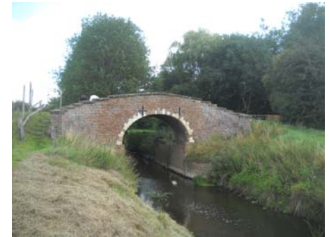
Plate 6 Strensall New Bridge
