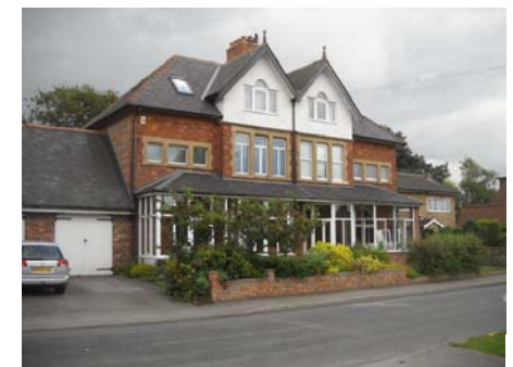
Plate 17 Nos. 9 & 11 Moor Lane
