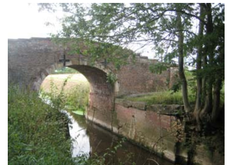
Plate 23 Strensall New Bridge
