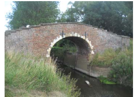
Plate 31 Strensall New Bridge
