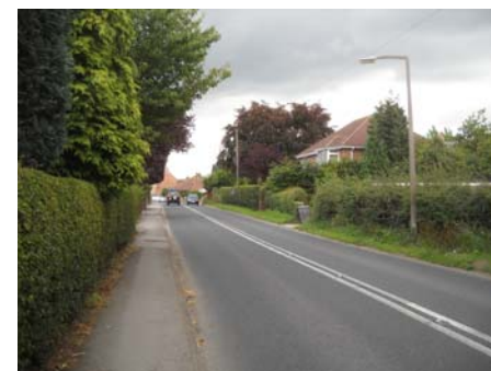
Plate 13 View north along York Road
