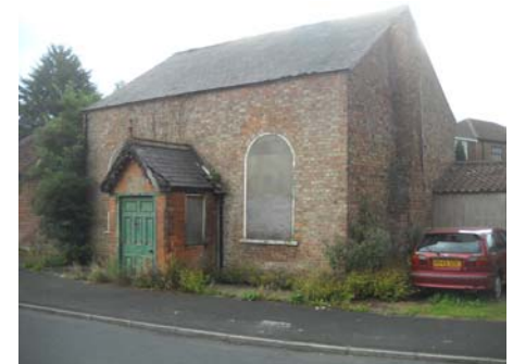
Plate 7 Former Chapel, Church Lane
