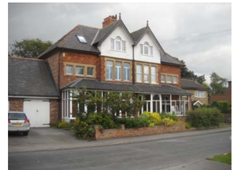
Plate 46 View of 9 & 11 Moor Lane
